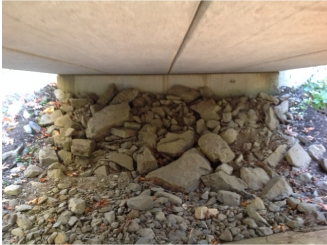
Left Bank Abutment when facing downstream
