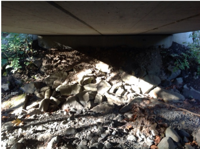
Right Bank Abutment when facing downstream
